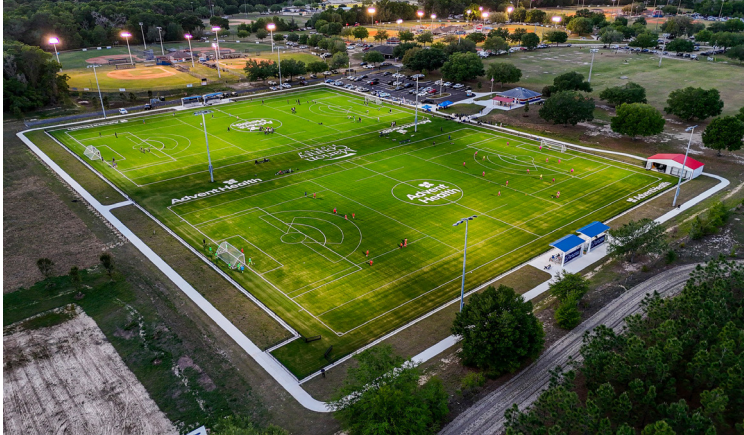
Ocala Rotary Sportsplex sports synthetic turf fields and upgraded infrastructure.
